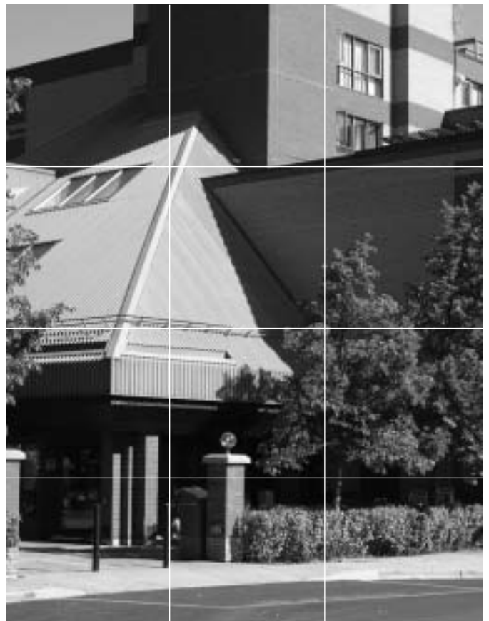
Safe-T-Element pilot project was conducted at the Peel Senior Link building – Manorbidge, Brampton
